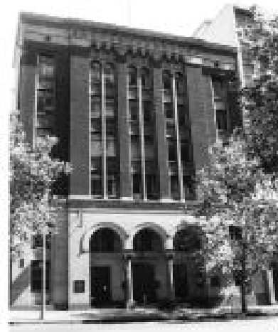
Equity Trustees Building, 472 Bourke Street, Melbourne (photograph courtesy J.T. Collins Collection, La Trobe Picture Collection, State Library of Victoria).
